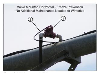
Figure 170-2 1. Aguamatic Valve 2. Plastic Tube
