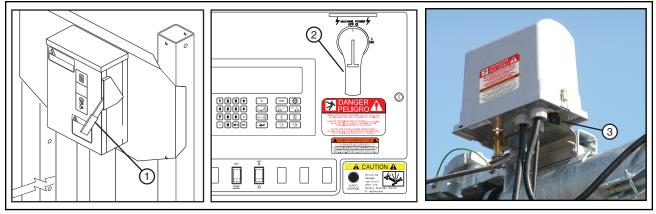
Figure 64-1 1. Main Service Disconnect Switch 2. Control Panel Main Disconnect Switch 3. Tower Box Disconnect Switch
