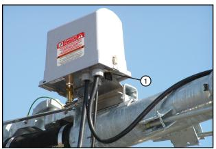
Figure 14-1 1. Disconnect Switch
