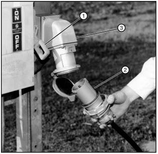
Figure 58-1 1. Service Disconnect - OFF 2. Power Plug 3. Receptacle
