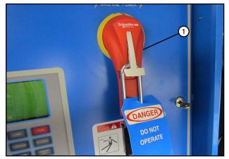
Figure 47-3 1. Main Power Disconnect Series 8000 Control Panel Shown
