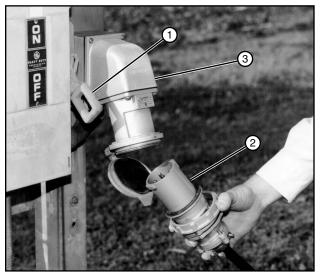
Figure 42-1 1. Service Disconnect - OFF 3. Receptacle 2. Power Plug
