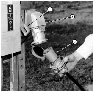
Figure 54-1 1. Service Disconnect - OFF 2. Power Plug 3. Receptacle
