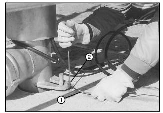
Figure 48-3 1. Ground Wire 2. Ground Lug
