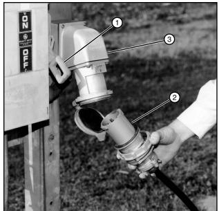
Figure 45-1 1. Service Disconnect - OFF 2. Power Plug 3. Receptacle
