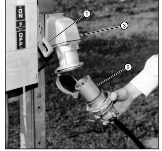
Figure 61-1 1. Service Disconnect - OFF 2. Power Plug 3. Receptacle
