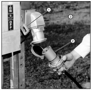
Figure 56-1 1. Service Disconnect - OFF 2. Power Plug 3. Receptacle
