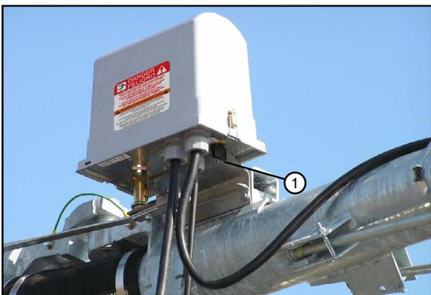
Figure 12-1 1. Disconnect Switch
