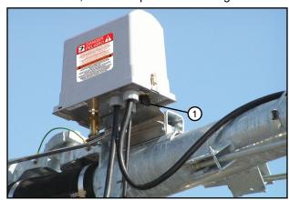
Figure 12-1 1. Disconnect Switch
