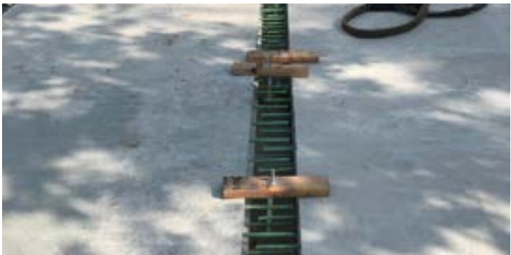
Deck joint prior to filling with T-17.
