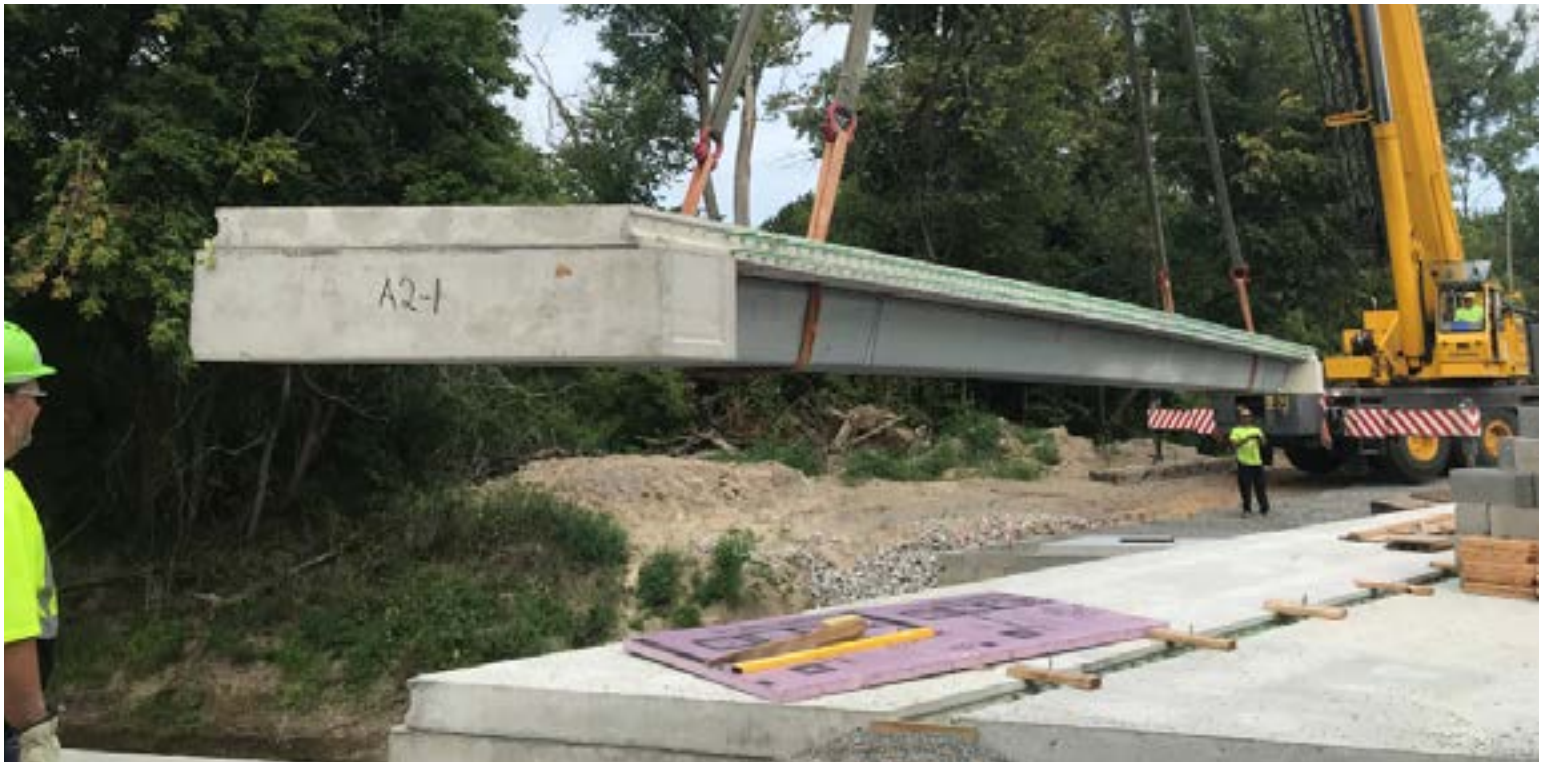
Valmont ABC bridge system being installed in Midland County, MI
