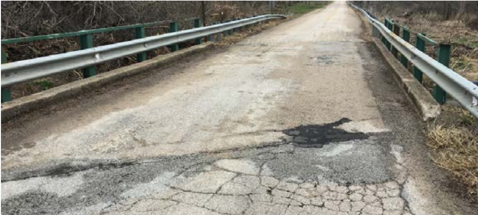
Existing deteriorated Orr Road Bridge.
