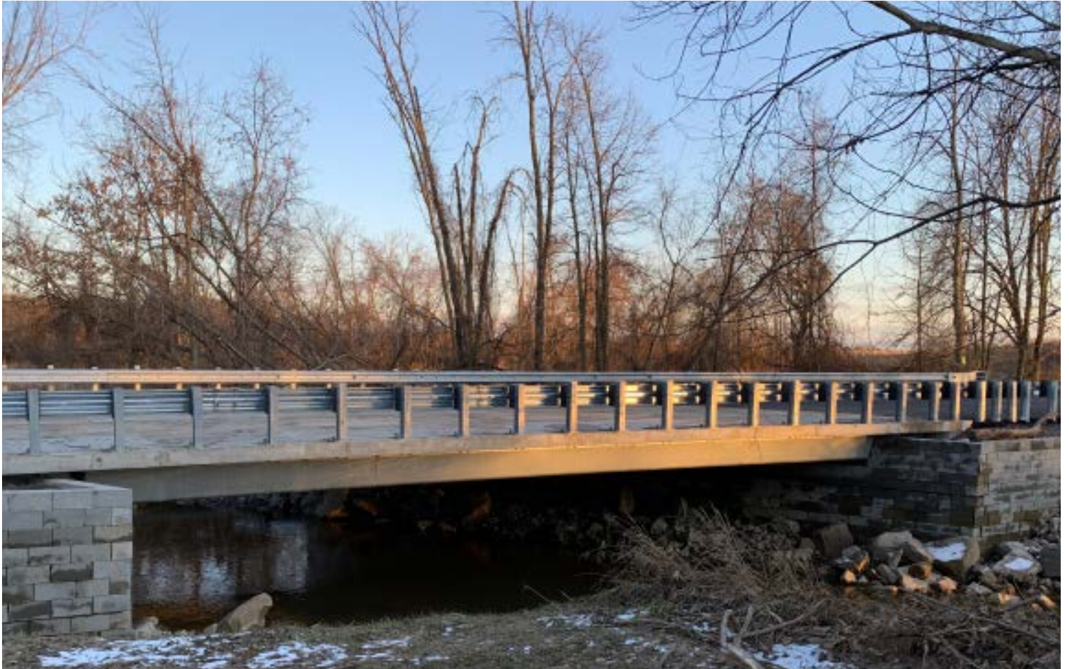
Valmont ABC bridge system on Geosynthetic Reinforced Abutments in Midland County, MI
