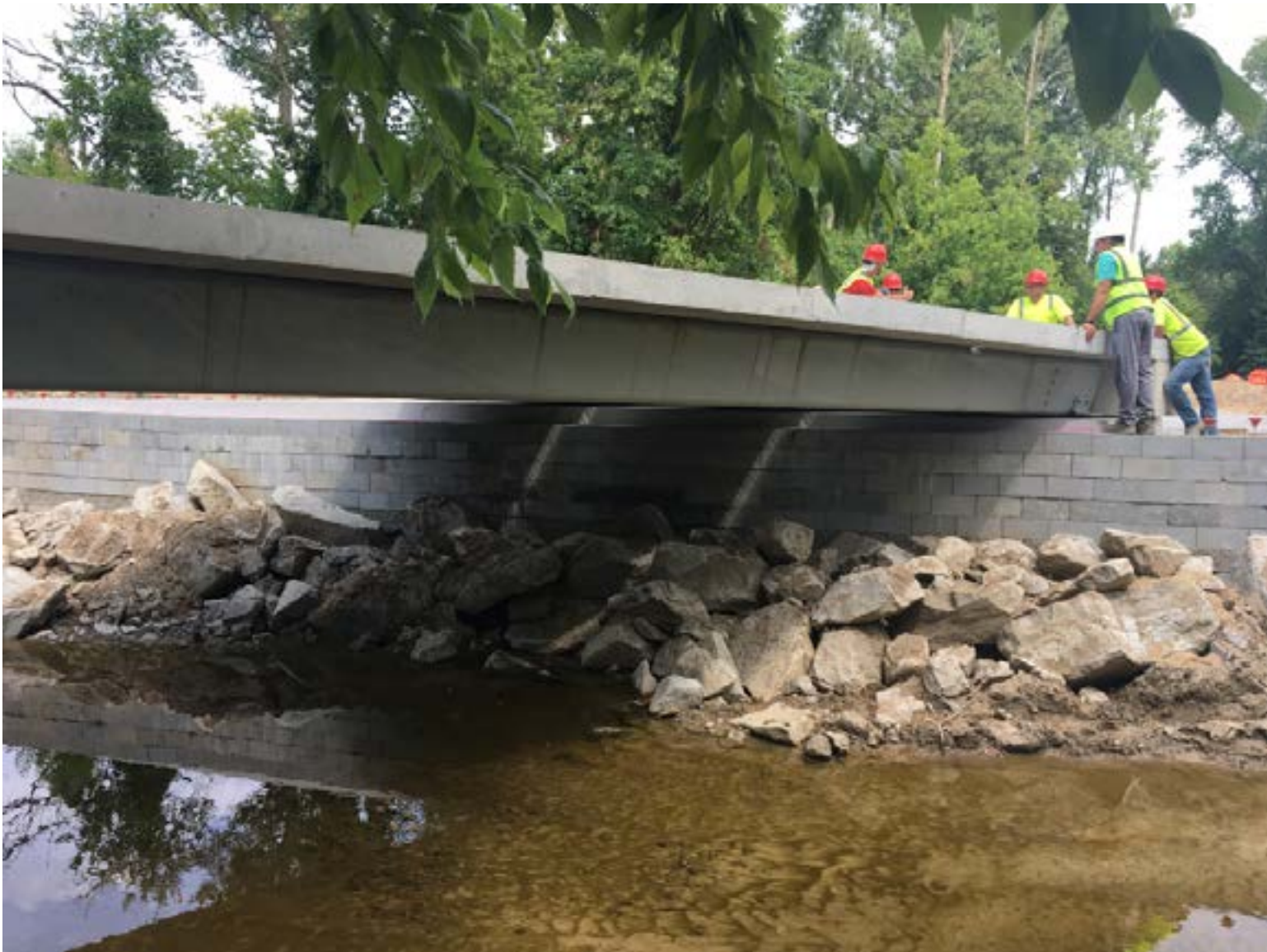
Valmont ABC bridge system being installed in Midland County, MI
