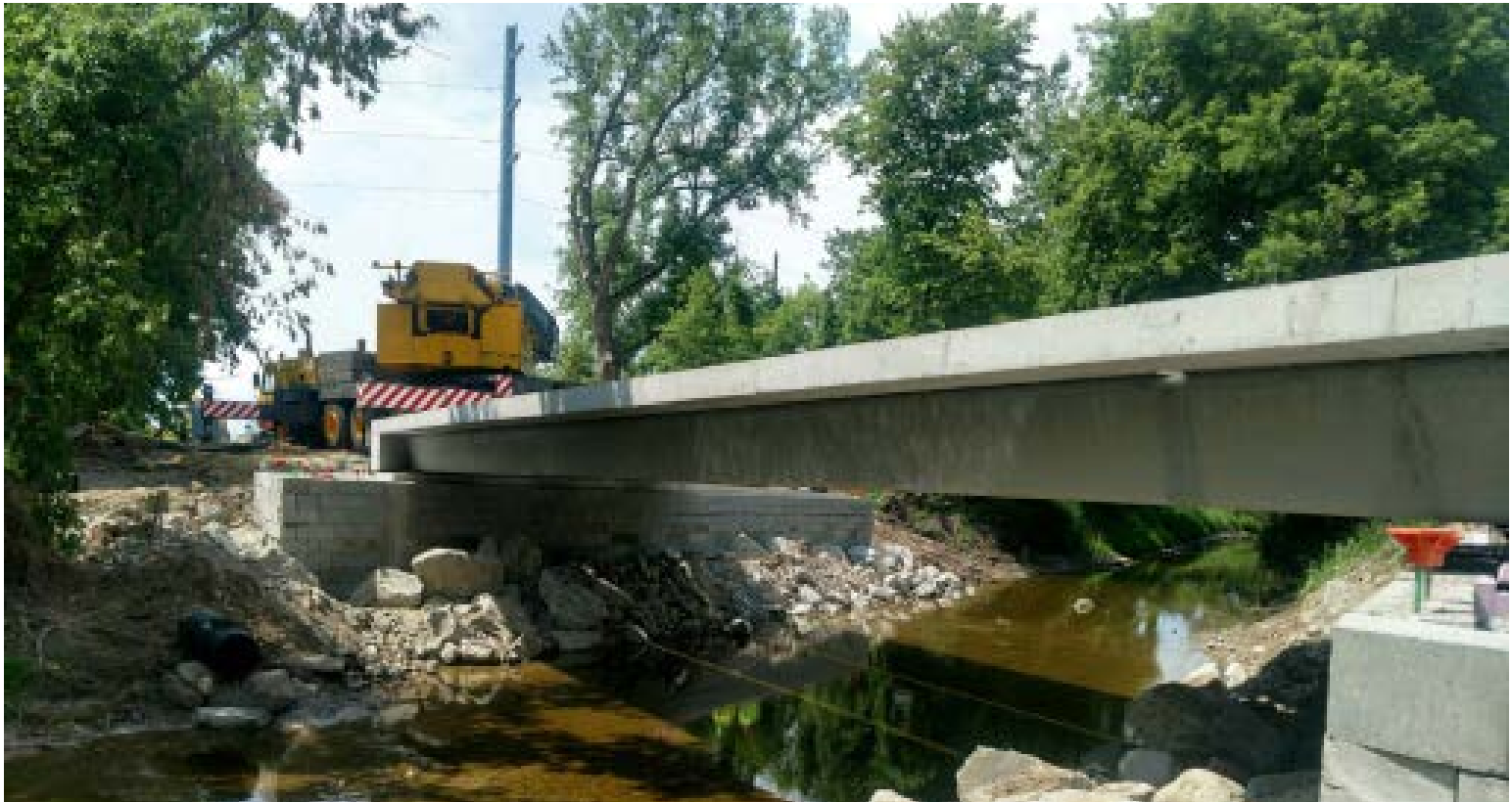
Valmont ABC bridge system being installed in Midland County, MI
