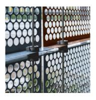
This project was to build a decorative facade and sunscreen that could also act as a pedestrian barrier for the new seven-level, 567-space parking building. In order to achieve greater installation efficiency and a more practical solution, we re-envisioned a design utilizing Atmosphere facade system after being approached by Thiess.
