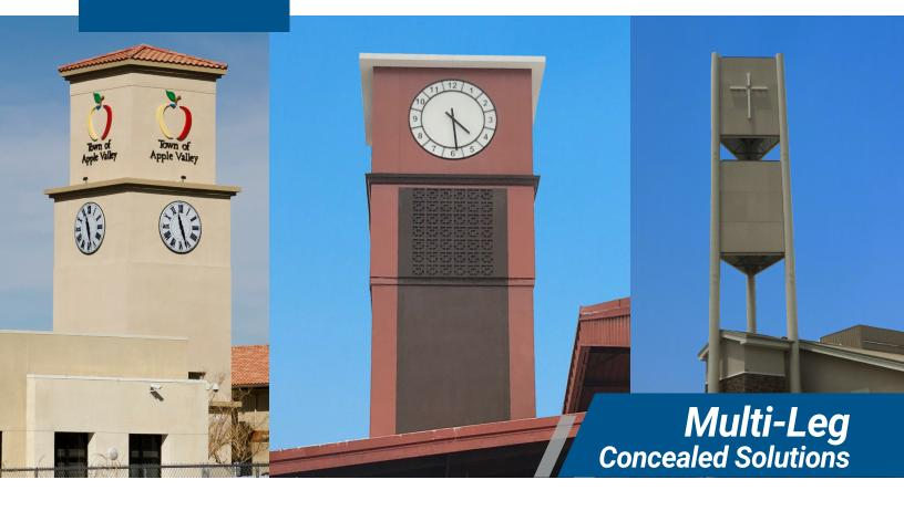
Valmont Larson offers a full line of marquis towers, bell towers, and clock towers as an option for multi-leg camouflage designs. As with most of our concealment structures, the ability to adapt is part of what we do best. Jurisdictional design challenges can be met with simple and reliable tower structures for multi-leg based products. Our RF-friendly materials are tested in a laboratory and in the field.
