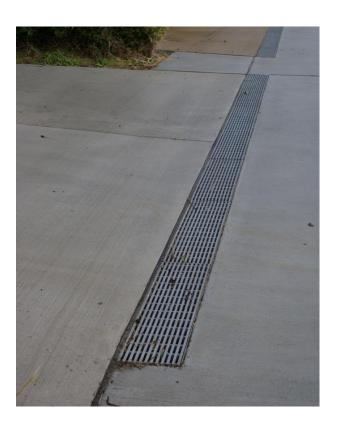
These photos show our 200mm clear opening drainage channels complete with locked down longitudinal heelguard grates after installation.
